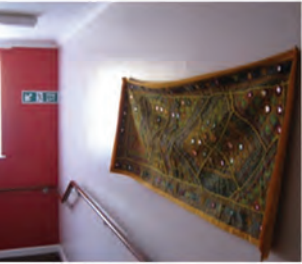
Flammable carpet on a wall can assist fire spread. Courtesy of Graham Fieldhouse.
