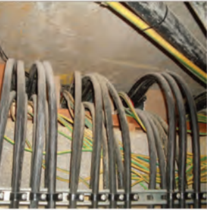
Power cables penetrating a compartment floor with no penetration seal installed (incorrect). Courtesy of Sharpfibre Ltd.
