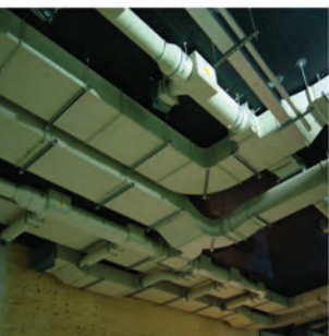
Installations of fire resisting ductwork. Courtesy of StGobain Isover (top) and Fire Protection Ltd (bottom)
