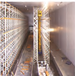
Tall buildings in warehousing/ food factories are often constructed from sandwich panels.
