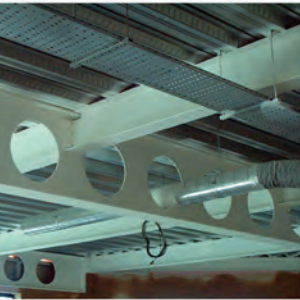
Cellular beam coated with intumescent paint.
