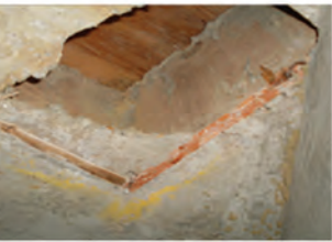
Compartment floor with a hole passing through to the laminate floor in the flat above (incorrect). Courtesy of Sharpfibre Ltd.
